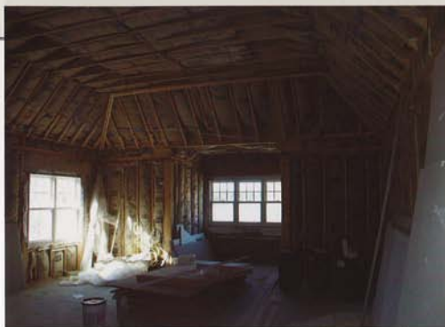
ABOVE: The interior room envelope is framed and insulated. The windows, though you can't see them in the theater, keep the balanced appearance of the exterior of the house.
