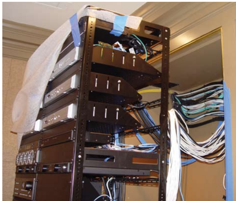
A closer shot of the rack before wire dressing.
