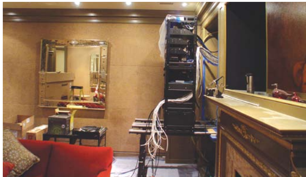
A shot showing the two of the four Middle Atlantic AXS racks after they arrived from testing at the AAT facility. The foreground shows the cavity for the former plasma as well as the track used to roll the custom art piece out of the way.
